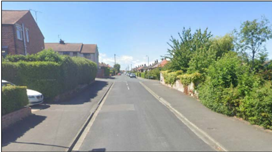
Plate TA4 - Section of Ffordd Pennant on Approach to Junction With Ffordd Gwilym / The Grove (note wide footways to both sides)
