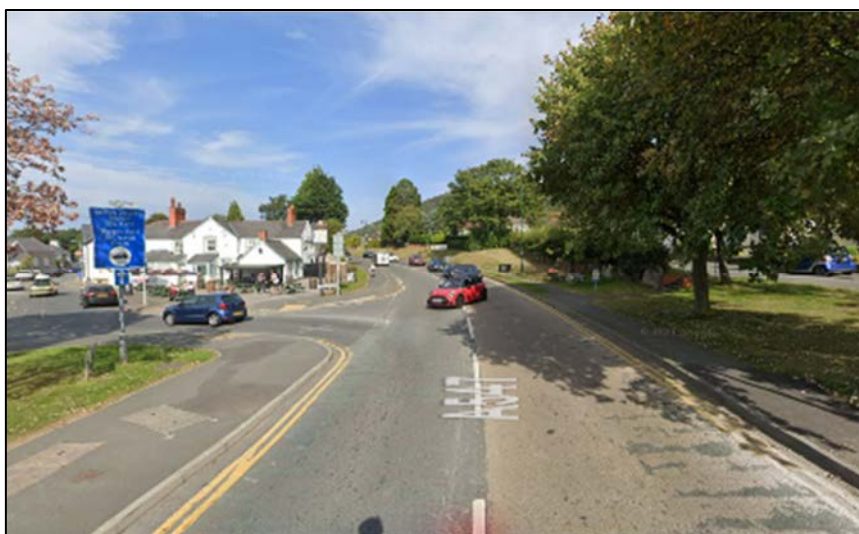
Plate TA9 - A547 entry junction to Ffordd Talargoch loop accessing Ffordd Penrhwylyfa
